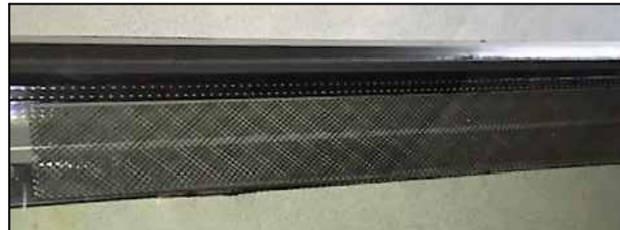
Photo as Viewed from Outside
